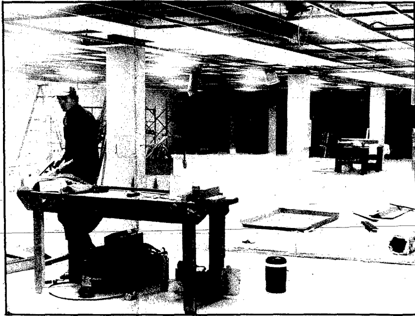
WORKMEN CONTINUE preparing the First National-Omaha Service Center facility for the start of operations in December.
